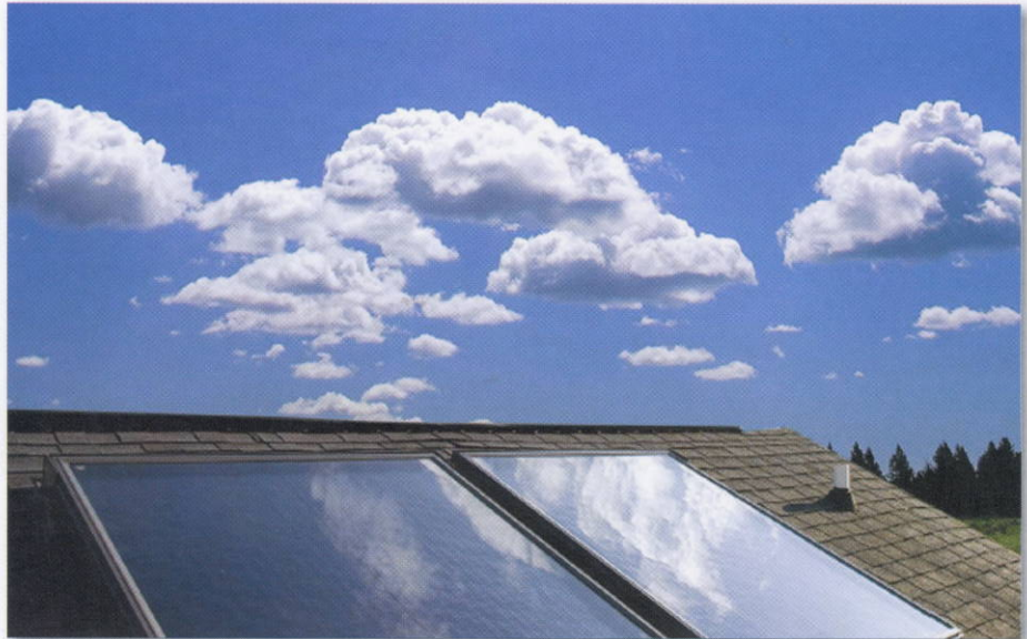
Velux, the Horsholm, Denmark based manufacturer of skylights and solar systems, has two facilities in Greenwood that employ more than 550 people.
