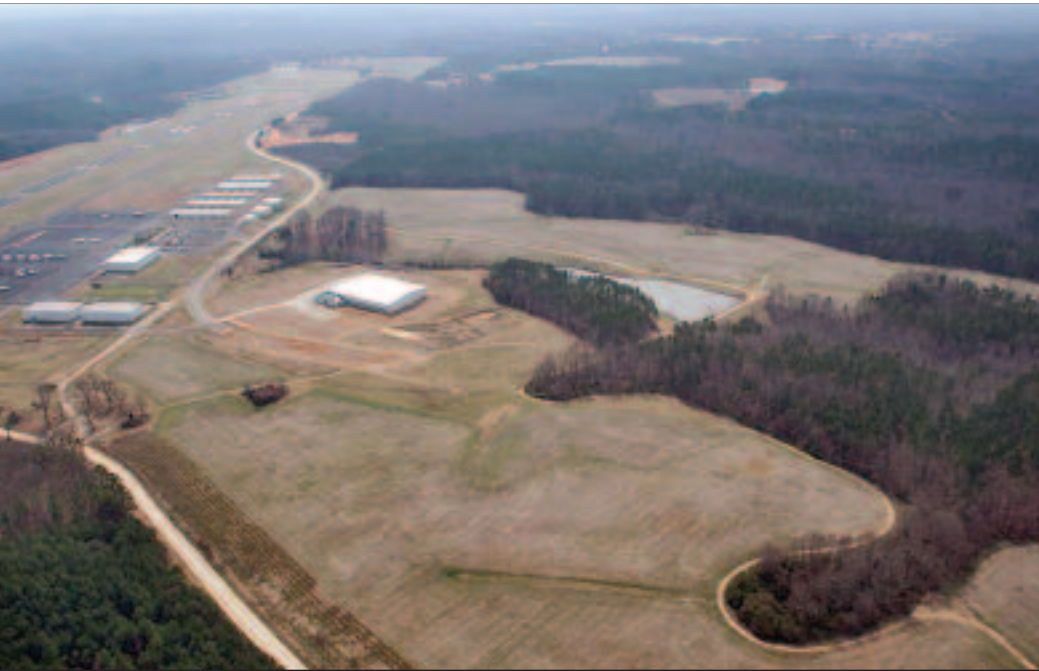
Triangle North Franklin is a 252-acre park that sits right next to Triangle North Executive Airport (top left). Its new building (center) offers 30,000 square feet for light industrial use and 3,900 square feet of office space. Aerial photo courtesy of Triangle North
